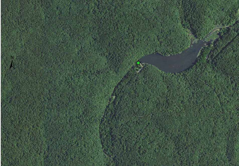
Figure 3.6. Noblett Lake Dam
